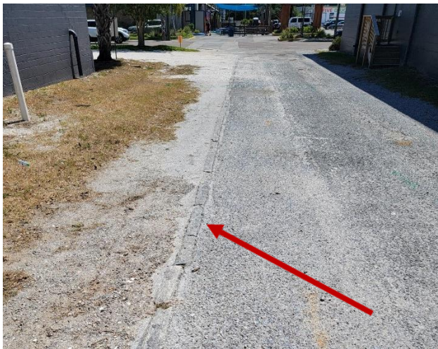
Figure 8. East end looking east toward 22 nd Street South. Photo shows granite curbing.
