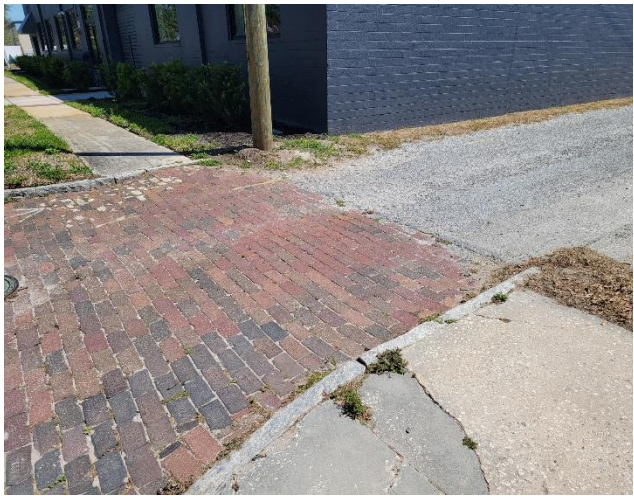
Figure 4. West end of alley looking north, brick and granite edge
