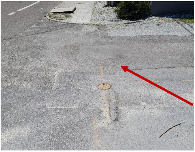
Figure 7. East end of the alley looking south, it is assumed that the historic brick underlies the apron but stops at the granite edge and does not extend along the alley.
