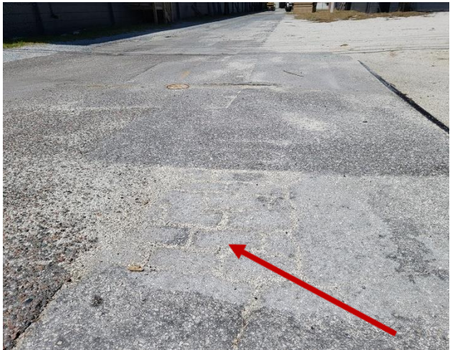
Figure 6. East end of the alley looking west, showing brick impressions underneath the apron paving.
