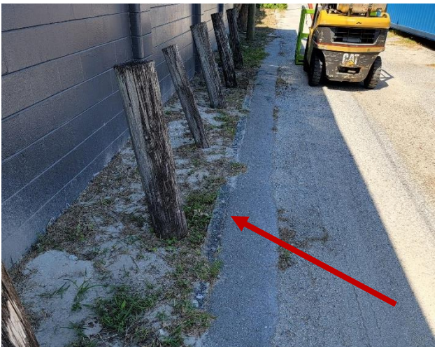
Figure 9. Center of alley looking west. Photo shows granite curbing.
